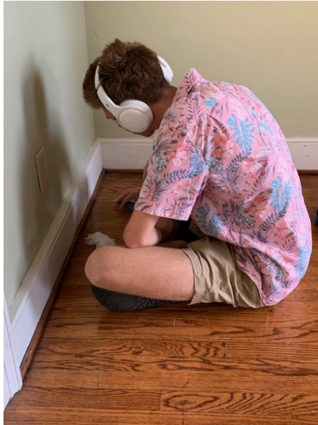
15-year-old Carter helps his grandfather remove paint splatters from the floor in Dr. Weir's office. (Fred Faust)
