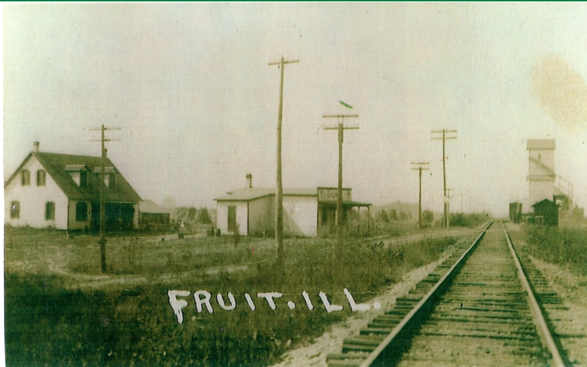
Undated photograph showing the intersection of Fruit Road and the Clover Leaf Railroad. The house at left still remains, but the "Saloon" in front (that's Fruit Road running in front of the saloon) has been gone for many years. On the west side of the track is the railroad station (the dark building) and the grain elevator. (Haarmann and Paproth)
