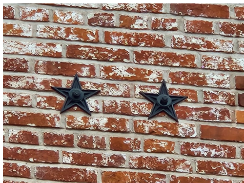
There are now four sets of these stars on the north/south walls of the Weir House.
