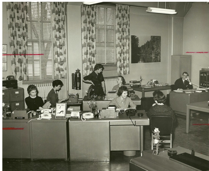
From a March 17, 1961 Edwardsville Intelligencer Telephone Special; “The business office at 119 S. Main will remain at its present location. Customer records are kept here, where the customer may pay his bill.”
