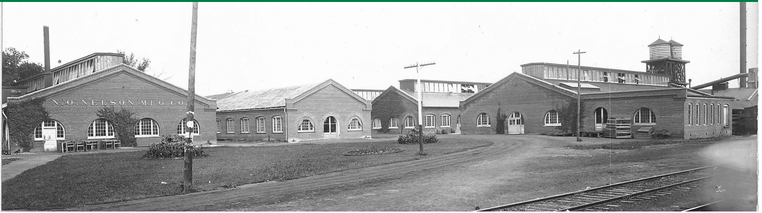
Undated photograph of the Leclaire factories, circa 1895. The line of clearstories along the roof allowed for light and ventilation. (MCHS)
