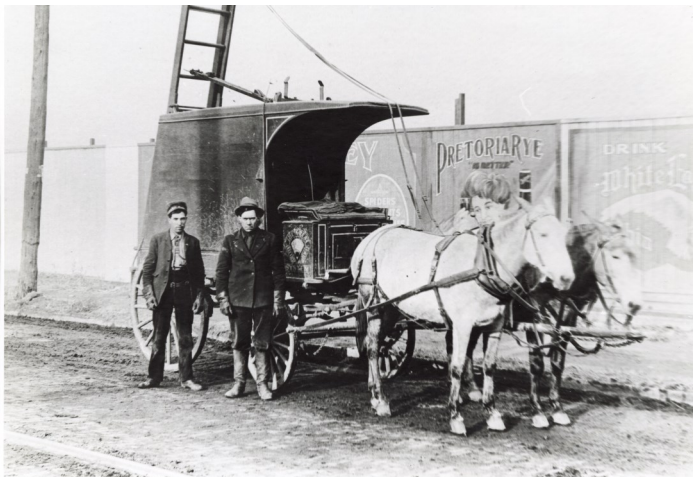
This horse-drawn line car in Alton was part of "The Great East Side Electric Railway System" whose logo can be seen on the side of the carriage and at right. Notice the ladder on the back which was used to repair the overhead electrical line. ( MCHS)
