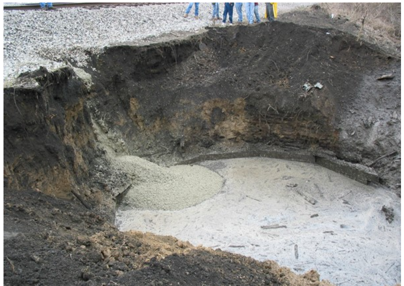
Figure 4. Shaft liner for the Henry Ritter Mine as seen during the AML Emergency Program remediation efforts taken to ensure public and railroad safety.
