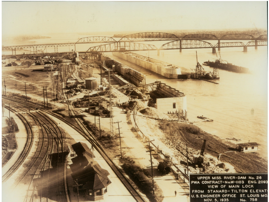
Construction of the first lock and dam at Alton in 1935. (Courtesy of Don Huber)
